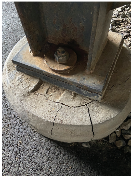
Fig. 5-9. Examples of rust jacking and cracking induced by oxidized embedded steel (photos courtesy of Simpson Gumpertz & Heger).
