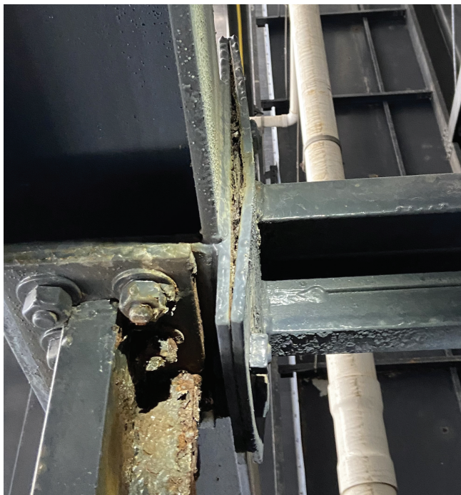
Fig. 5-9. Examples of rust jacking and cracking induced by oxidized embedded steel (photos courtesy of Simpson Gumpertz & Heger).
