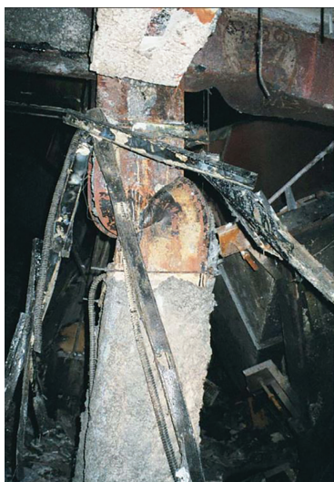
Fig. 6-1. Examples of fire-exposed beams and columns from FEMA (2002).
