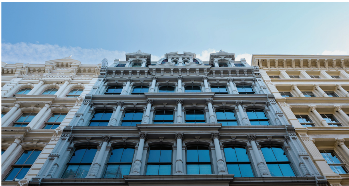
Fig. 4-2. Historical ornamental cast iron facades in SoHo, New York, N.Y. (photo courtesy of WireStock).
